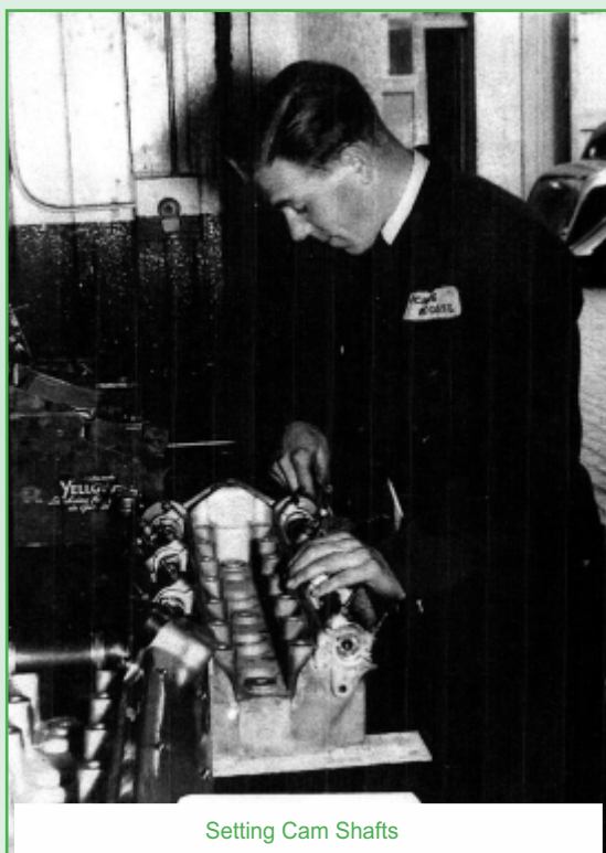
1956 3.8lt 'D' Type Engine with Lucas Fuel Injection & wide angle head.
